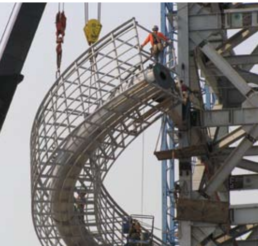
Steel being erected for the theater tower.
