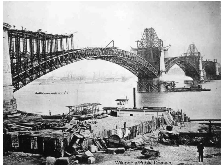
Construction of the Eads Bridge crossing the Mississippi River at St. Louis, Mo., around 1874.
