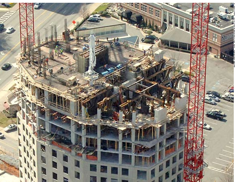
The slab is being formed on the south side of the tower as truss erection continues on the north side. Integrated steel truss erection with slab placement minimized the schedule impact of on-site truss erection. The only way to transfer the column loads resulting from stepping the building in was to use structural steel transfer trusses that are the full depth of the floor.
