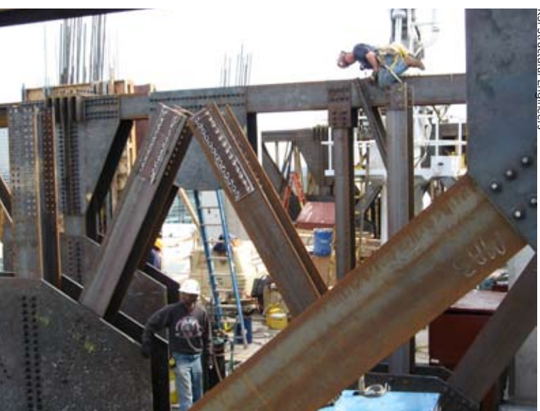
To keep from having to use a larger crane, the transfer trusses were lifted into place in pieces each weighing 22,000 lb or less, which were then bolted together using 14,200 high-strength bolts (in addition to the 5,700 used in the shop).
